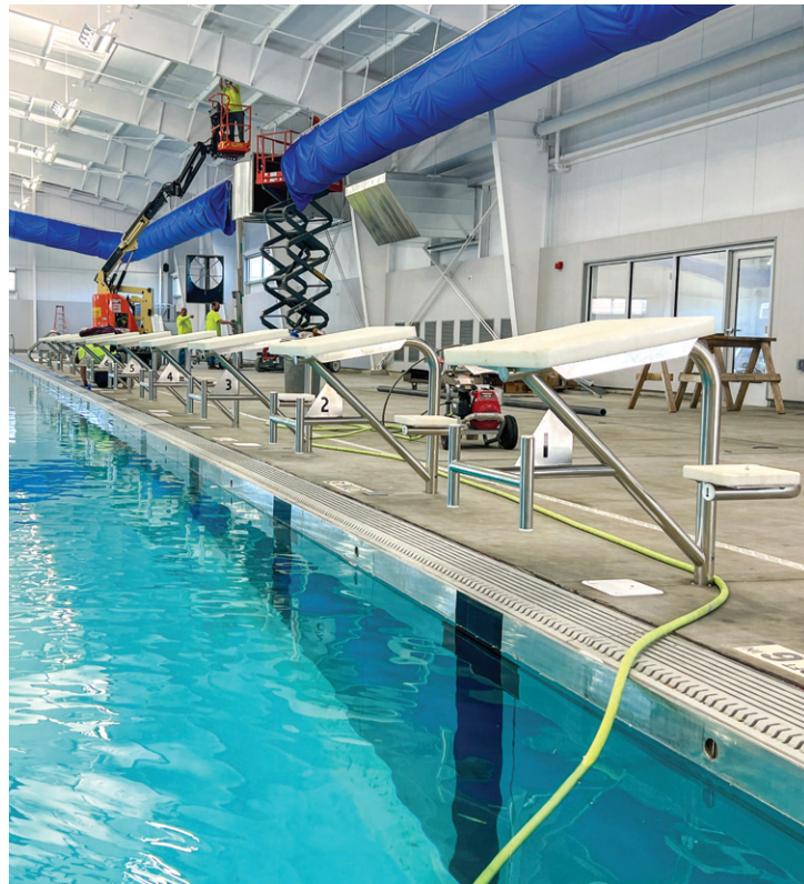
Stop by to see the newly renovated Cape Aquatic Center!
